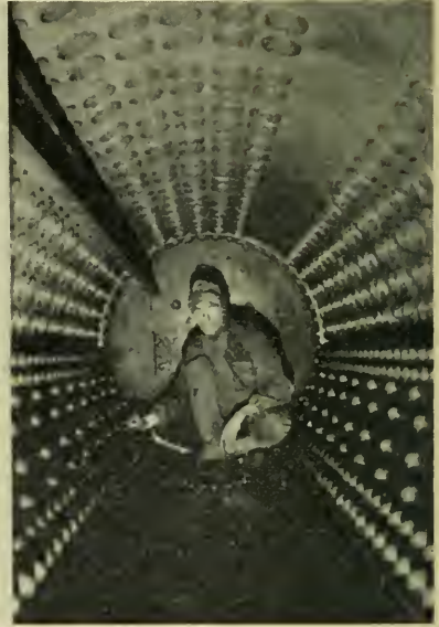
Exterior and interior views of boiler drum repaired with extra-wide straps to overcome weakness caused by caustic embrittlement.
